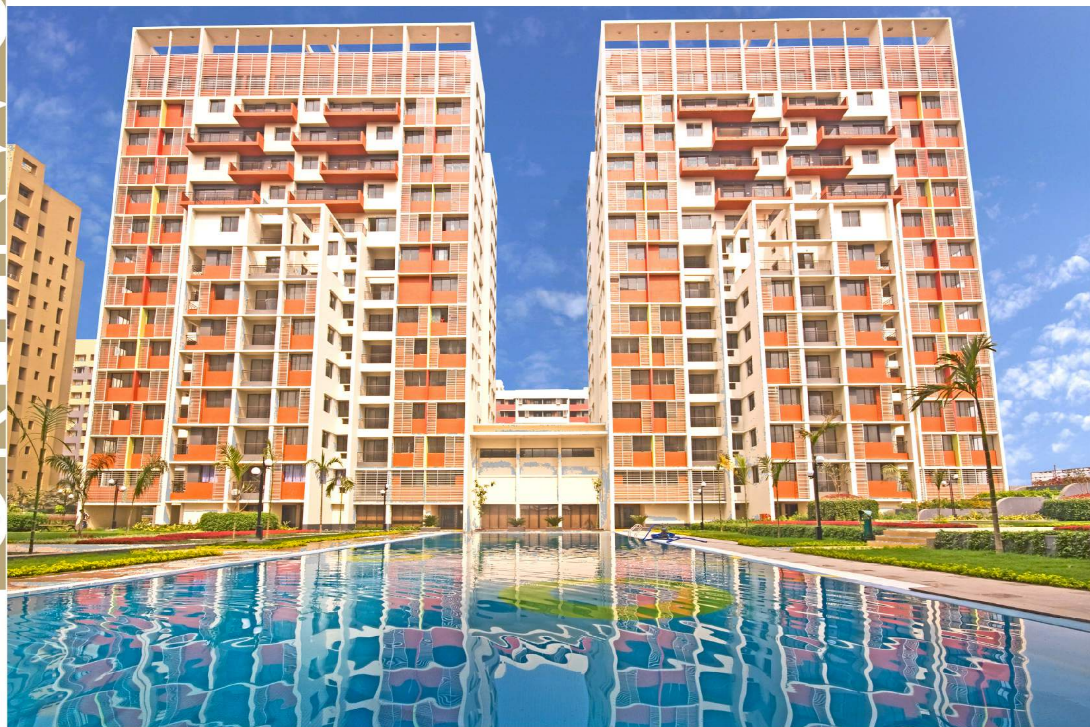
VIEW OF HIG TOWERS FROM SWIMMING POOL
